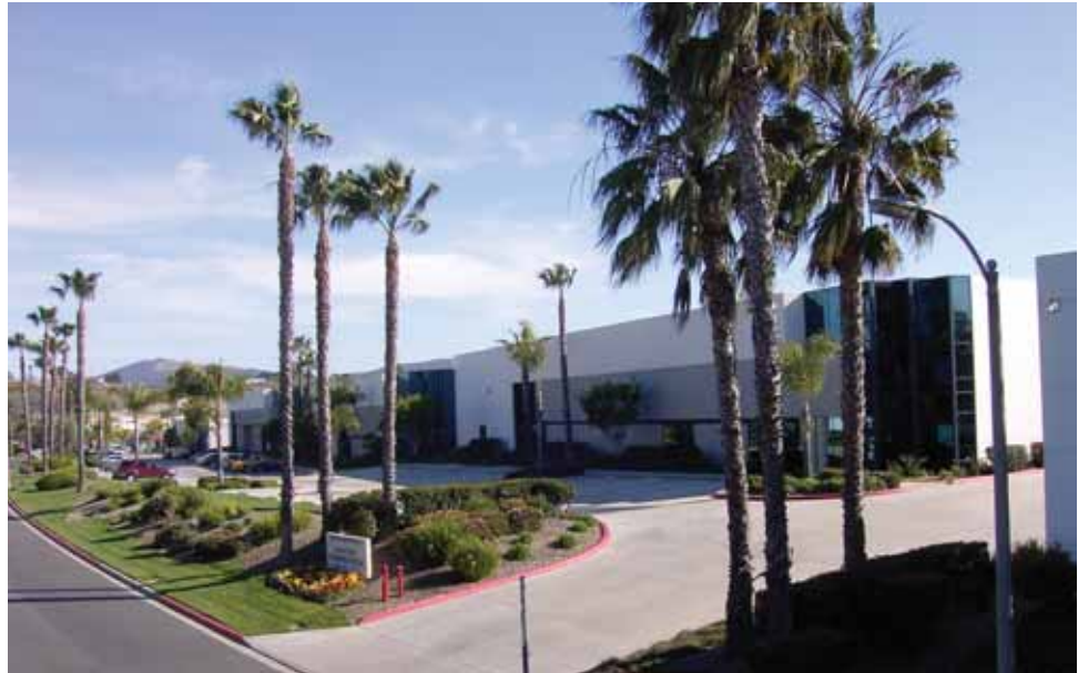
West Coast Distribution Center
