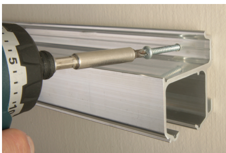
Step 1: Install wall-mount track.
