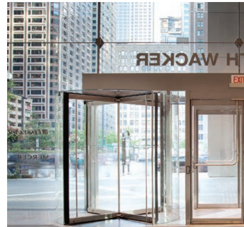
Crane SS4000-M (Complete Entrance) 155 North Wacker Drive, Chicago, IL Architect: Geottsch Partners LEED Gold Certified
