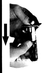
WARNING: Check alignment of latch hole center on the door and strike center on the jamb if resistance occurs against latch bolt movement of locking and unlocking. DO NOT USE EXCESSIVE FORCE OR TOOLS TO DRIVE THE LATCH
