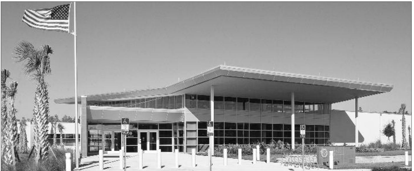
Project: Orlando Immigration Center, Orlando, FL
