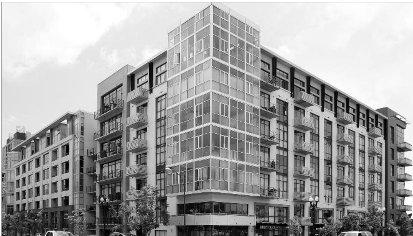
Project: M2i Lofts, San Diego, CA
