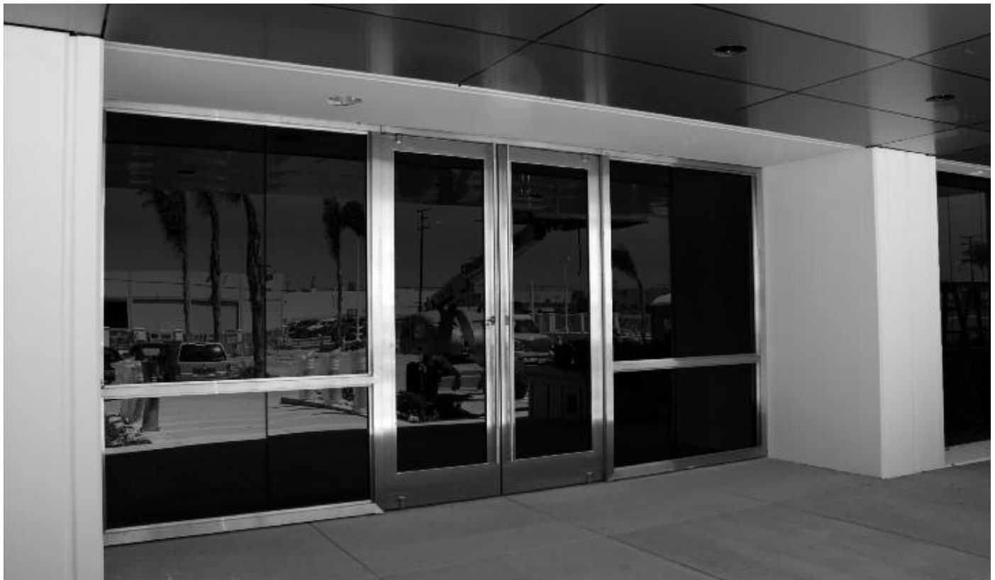
Project: Corporate Building Entrance, Los Angeles, CA
