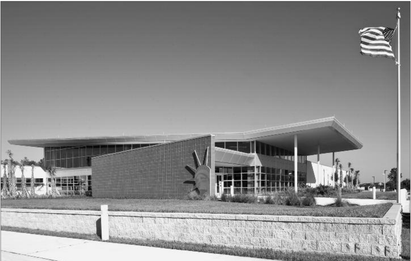
Project: Orlando Immigration Center, Orlando, FL
