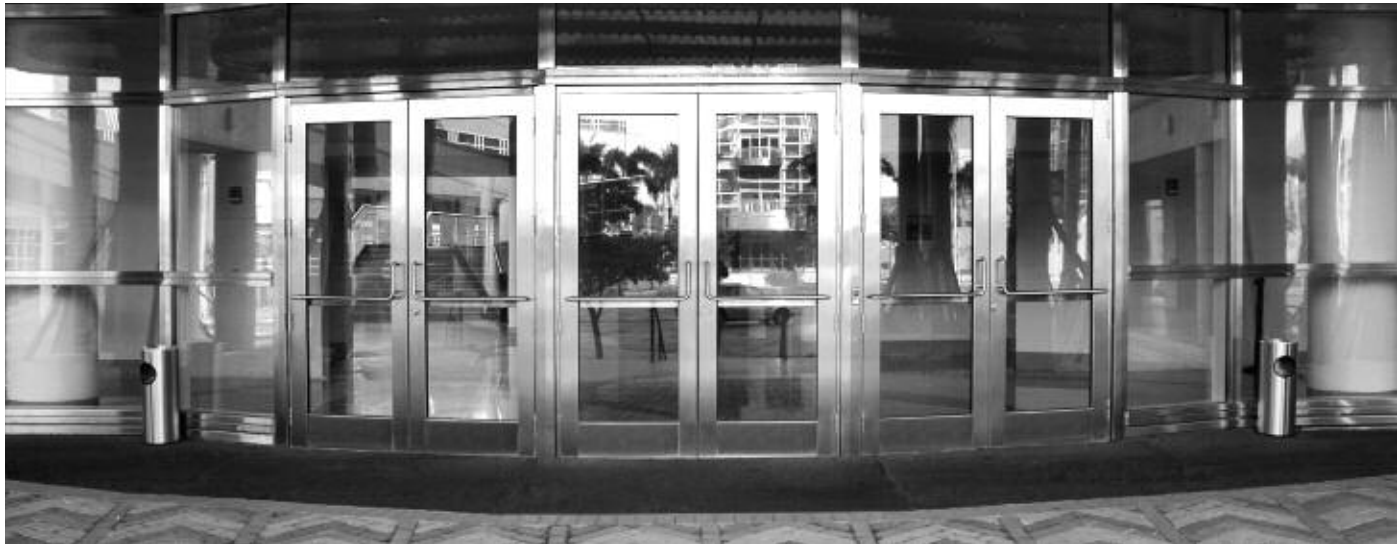
Project: Adrienne Arsht Center for Performing Arts, Miami, FL
