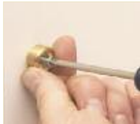
Set Threaded Insert to Wall
