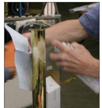
Clean Post for Installation
