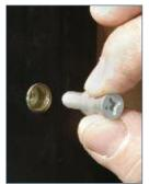
Lastly, insert the screw or bolt into the Rivet-Nut and tighten. The door stile is now ready to receive a Push/Pull Handle.
