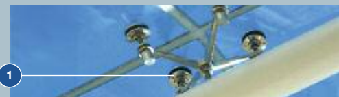
08 4426.19 – CRL Spider Fitting Point Supported Glass Awning System
