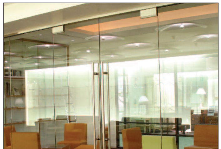
Overhead Concealed Closer used with Patch Fittings
