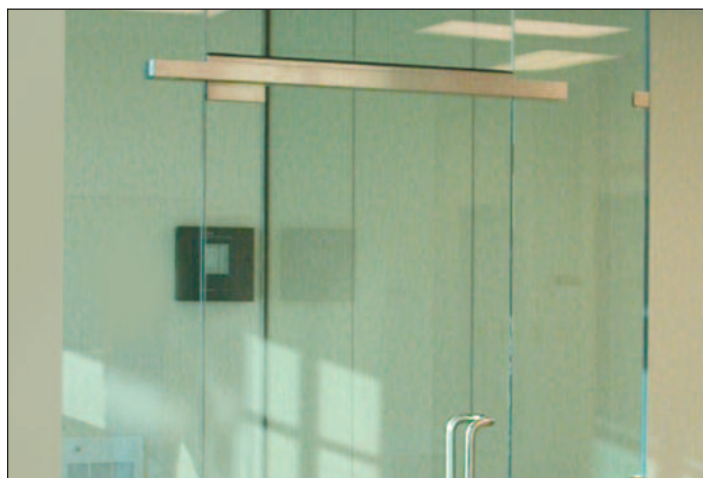
Overhead Concealed Closer used in a Floating Header
