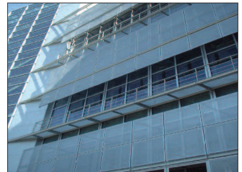
Typical Perforated Panel Detail
