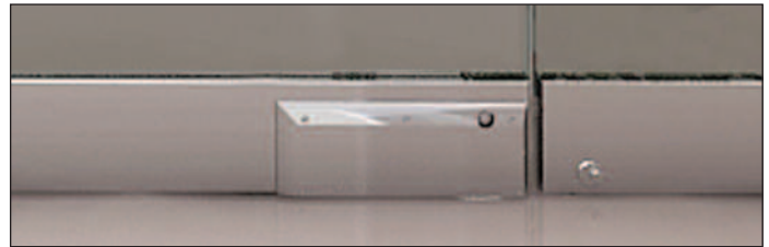
Heavy-Duty Floor Closer and Engagement Mechanism Concealed in the Bottom Rail
