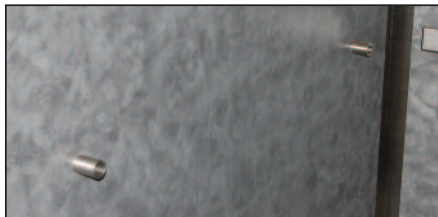
Secure Mounting Studs to Wall with Appropriate Fasteners
