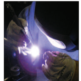
Welding on All Diameters
