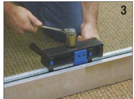
3 Tighten the TAPER-LOC® components using our measured Torque Wrench and you are done.
