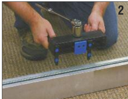
2 Place the TAPER-LOC® Installation/Removal Tool into position directly over the Taper Set.
