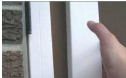
Vinyl screen doors incorporate a hinge bar, which eliminates the need of trimming to fit.
