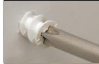
STEP 2: Press into gypsum wallboard while turning clockwise until seated flush with wall.
