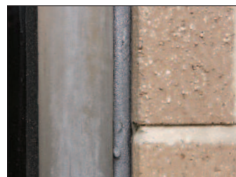
Insertion with sharp putty knife will tear "skin".
