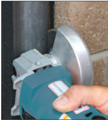
Mechanical Abrasion with Cat. No. 9553NB and LAB450
