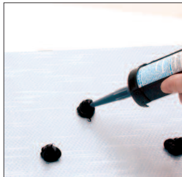
Applying mastic to mirror with Category II Tape applied to back with no holes cut out
