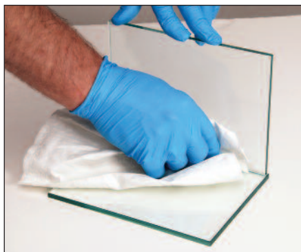
6. Remove Fixtures and Clean Off Excess Adhesive
