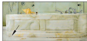
Installation Using Translucent White Silicone Sealant
