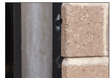
Out-gassing through torn "skin" will form bubbles in sealant!
