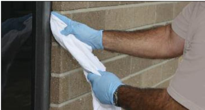
"Two-cloth" method - final wipe before solvent evaporates.
