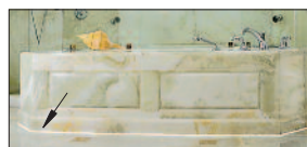
Installation Using White Silicone Sealant
