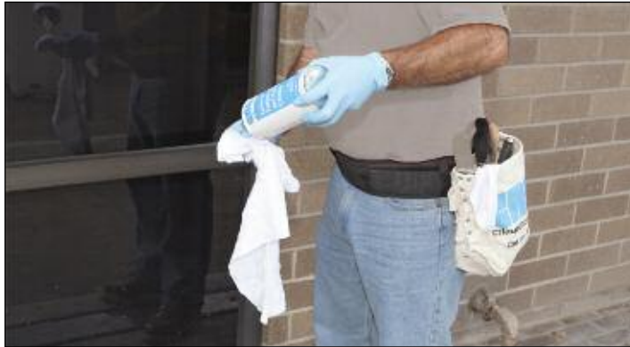
The Correct method is to pour on the cleaner. Dipping the rag into the solvent is incorrect, as this will contaminate the cleaning agent.
