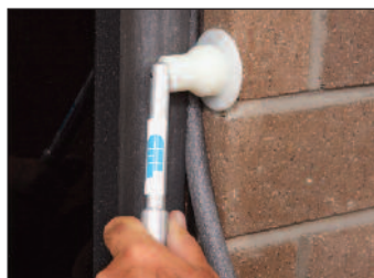
Cat. No. SBRR Roller Tool will not tear "skin" of Backer Rod.
