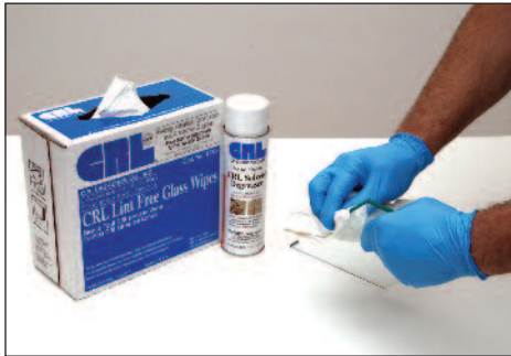
First, clean the edges to be bonded with Cat. No. CRL7528 Cleaner and Degreaser and Cat. No. 1550 Lint Free Glass Wipes
