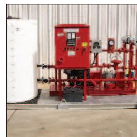
Diesel Pump Skids
