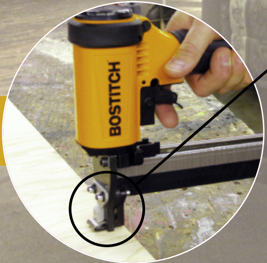
438S5 Stapler applying anchor clip to chair rail
