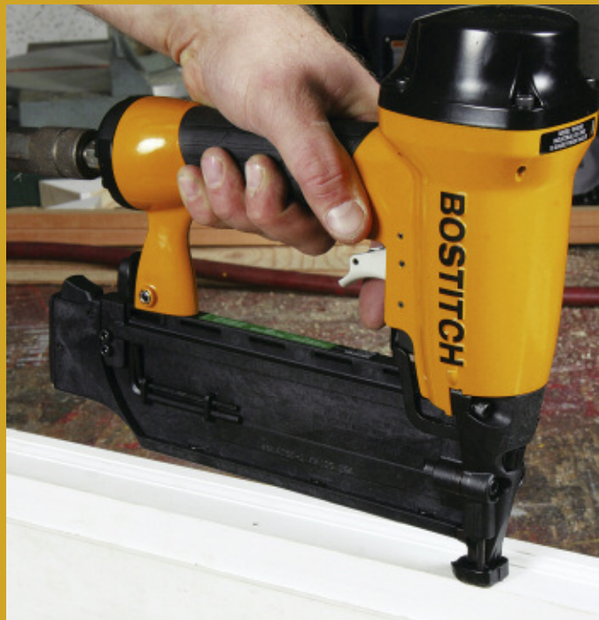
16-gauge finish nails connecting brick molding to a window frame
