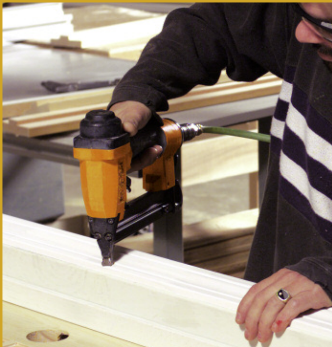
Applying 18-gauge brad to door casing
