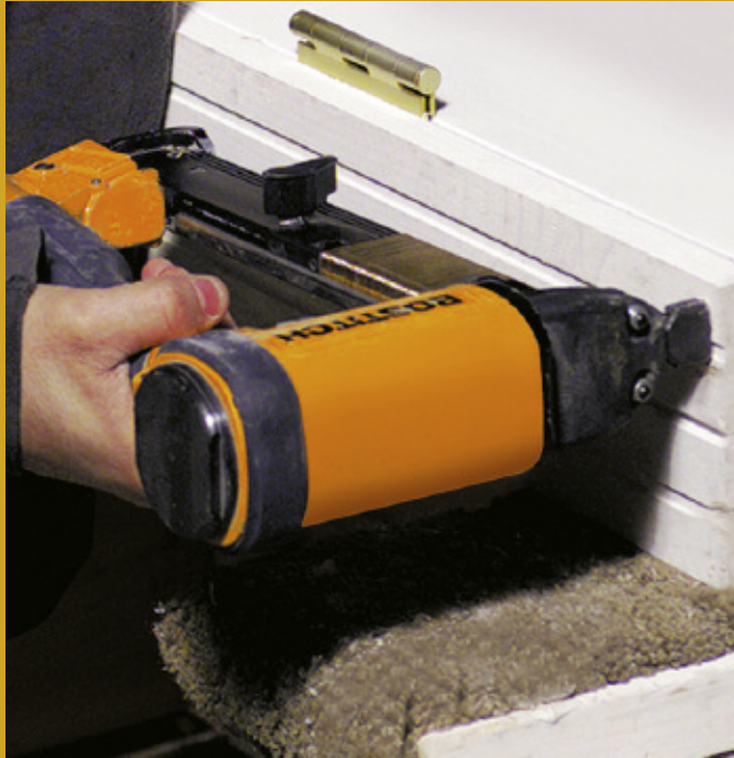
450S2 Stapler joining door jambs
