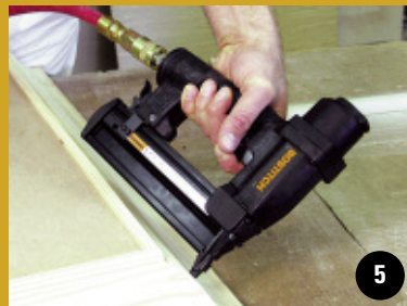
18-gauge brads applying trim
