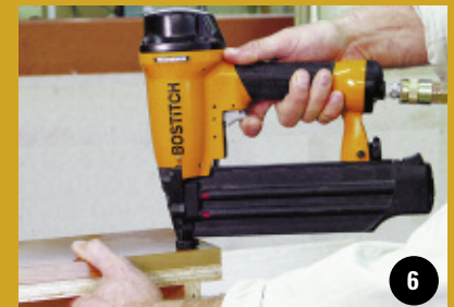
16-gauge nails securing a cabinet face
