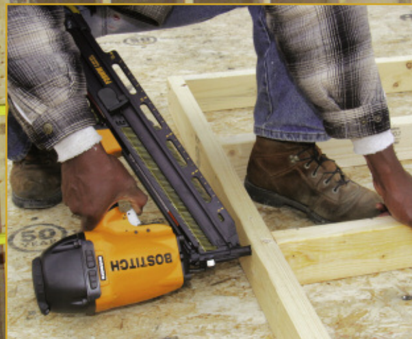
F28WW Assembling 2" x 4" stud wall
