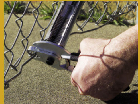
HFP9 Attaching tensioning wire to chainlink fence with 9 gauge aluminum hog rings
