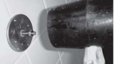
14. Verify the length of the nut from the *WingIt*<sup>TM</sup> faceplate is correct (step 8) – Then hit the *WingIt*<sup>TM</sup> firmly with a rubber hammer.
