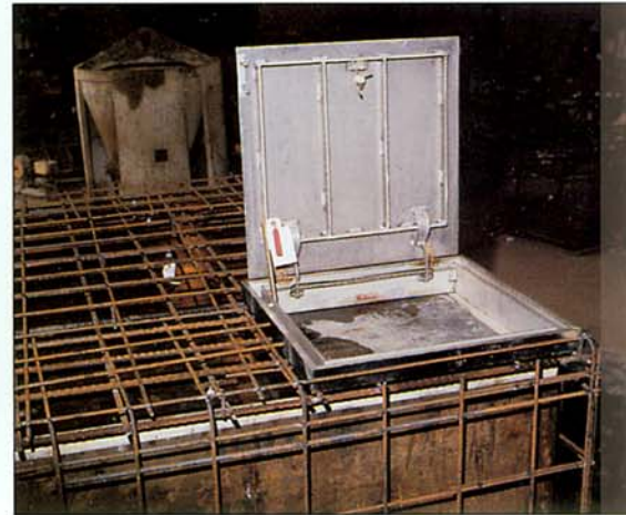
Frame depth designed to match slab thickness
